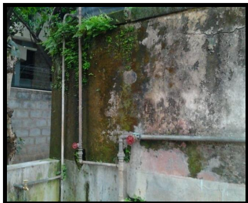
Figure 1: Microbial activities on domestic building at Haridwar (Uttarakhand)
